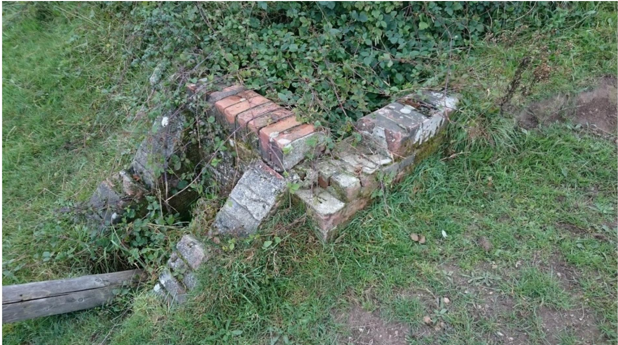
Plate 4: Old brick structure, potential drainage feature.
